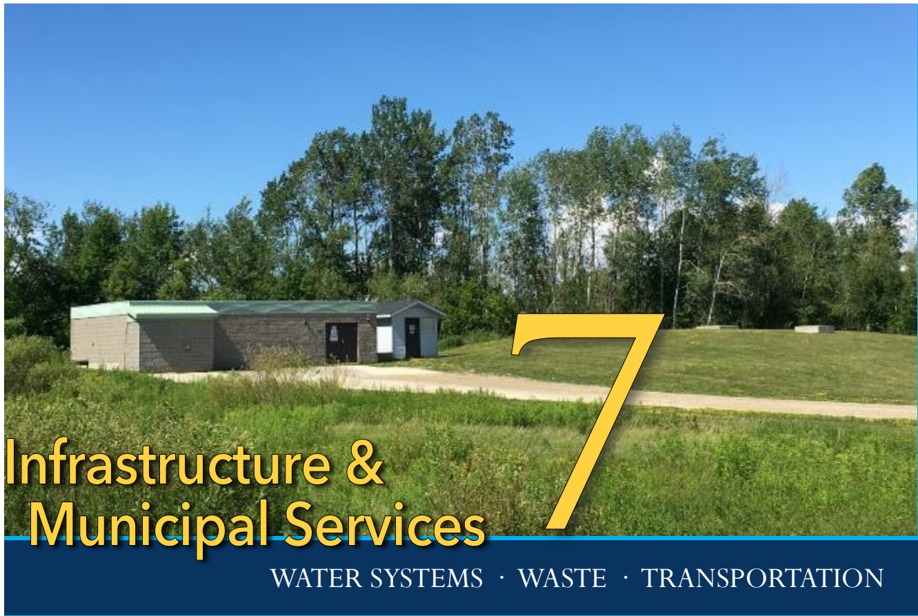
Photo: Water treatment plant in New Lowell Recreation Park.
